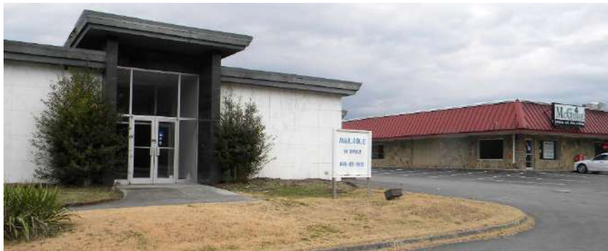
This vacant bank building is one of many vacancies in the area.
