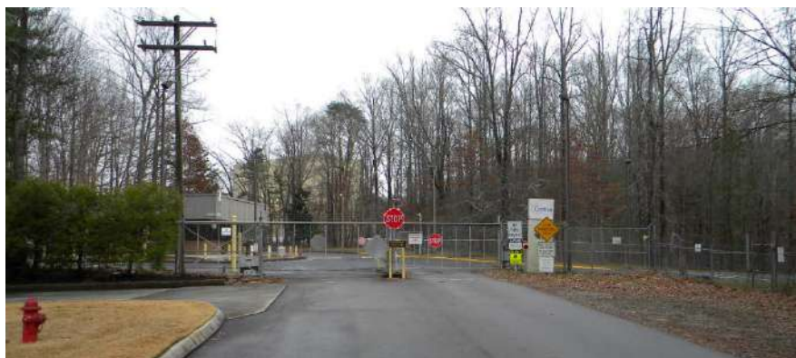
Mitchell Road terminates at a secured site.
