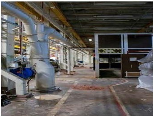
Alpha 5 Facility, post-Recovery Act cleanup effort. (2011)
