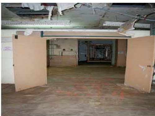
Alpha 5 Facility post-Recovery Act cleanup effort. (2011)
