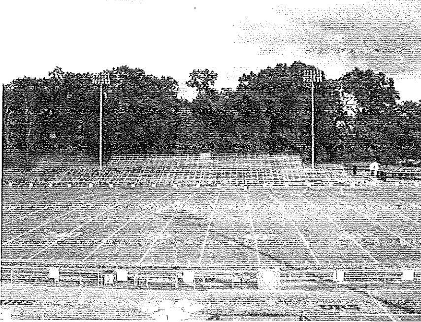
Photo 1: Visitor's (East Side) Metal Bleachers – View Looking East
